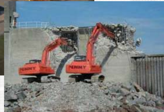
Final site clearance
